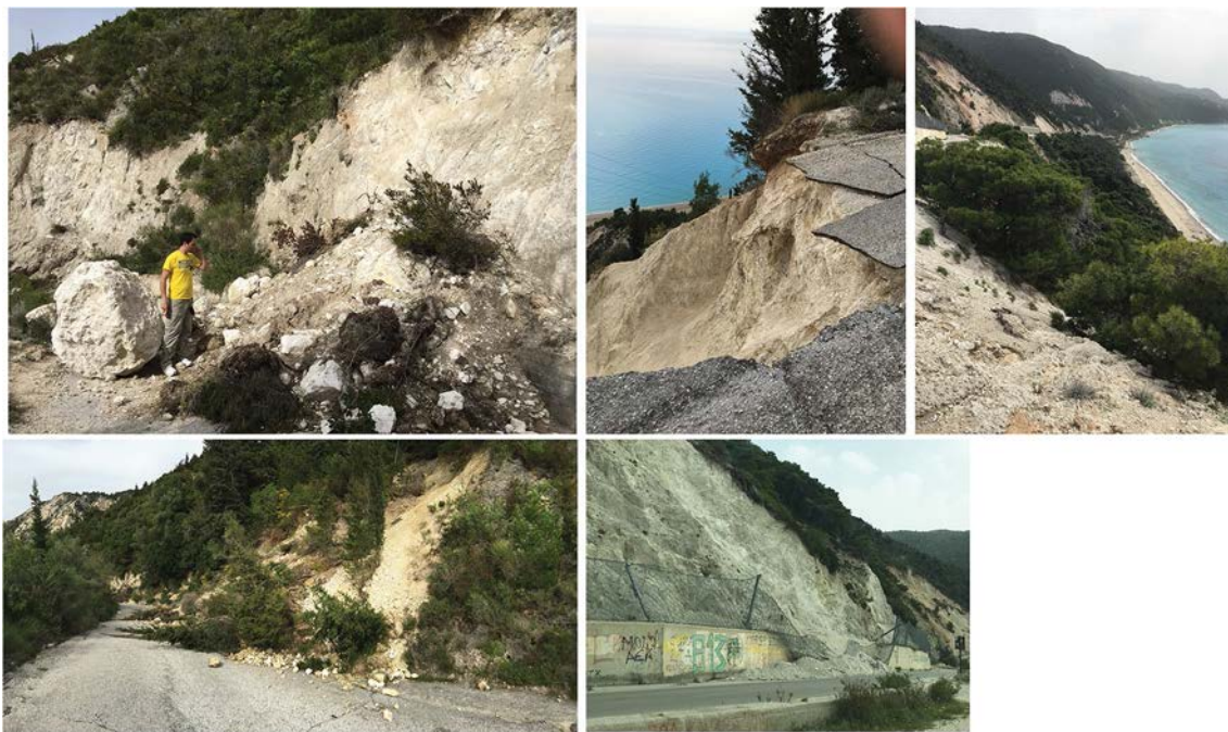
Fig. 8 Field perspective of volume loss over landslide regions
