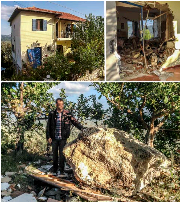
Figure 1. View of the rock block, the house it impacted near the end of its trajectory and the damage to infill walls that it caused.
